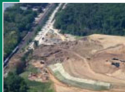
Disturbing slide prone Pittsburgh Red Beds and altering the hydrology of this site are two possible causes of the Kilbuck landslide.
